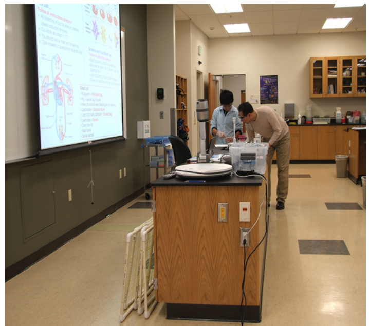
Students work on lab projects in a biology class at Skyline College. The AV cabinet houses connections to equipment as well as the SP Controls Pixie, which is used to operate the ceiling mounted projector.
